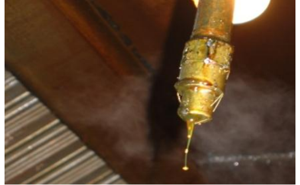
Grease, created by deep fryer cooking, dripping off a fire suppression nozzle
