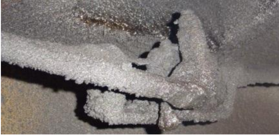
Grease has completely encased the detection and distribution components. Additionally, this system is improperly installed. The nozzle location will interfere with the ability of the fusible link to detect heat rise.
