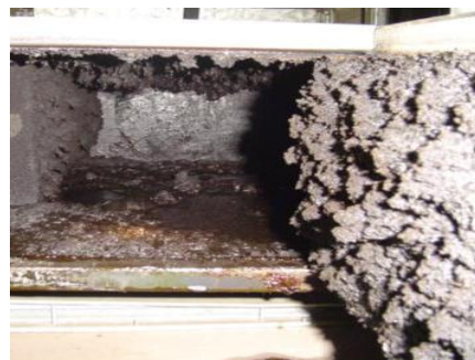
Looking into a duct opening found in the suspended ceiling. The access panel is on the right. Primary accumulation of gas charbroiler.
