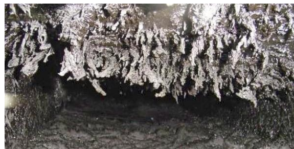
Examples of grease created by solid fuel charbroiler cooking
