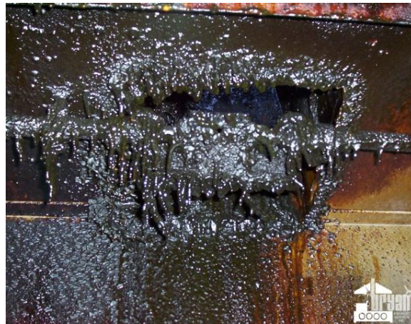
A completely impacted extinguishing system in the plenum of an oriental kitchen. Courtesy of Bryan's Exhaust Cleaning.
