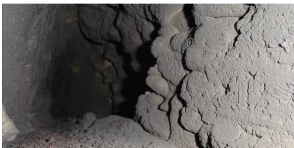
Examples of grease created by solid fuel charbroiler cooking
