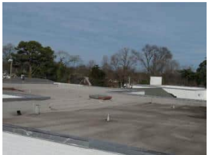
49. Low-sloped built-up roof assembly at Building 2109.
