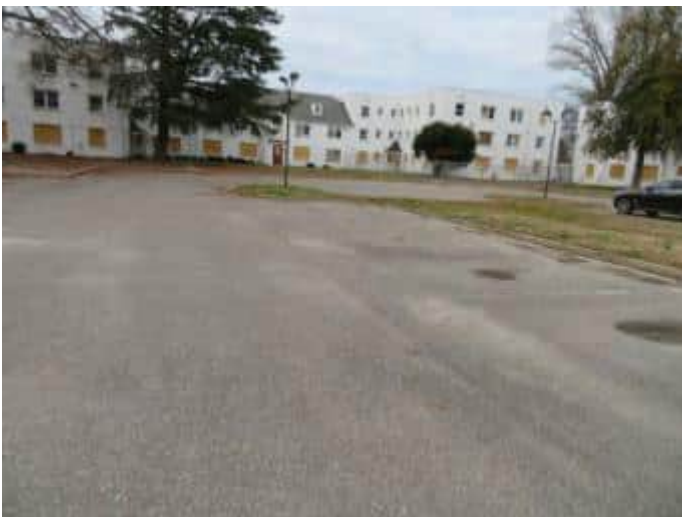
3. Typical condition of asphalt pavement.
