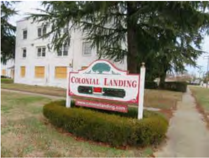
20. Monument signage at the entrance to the site.
