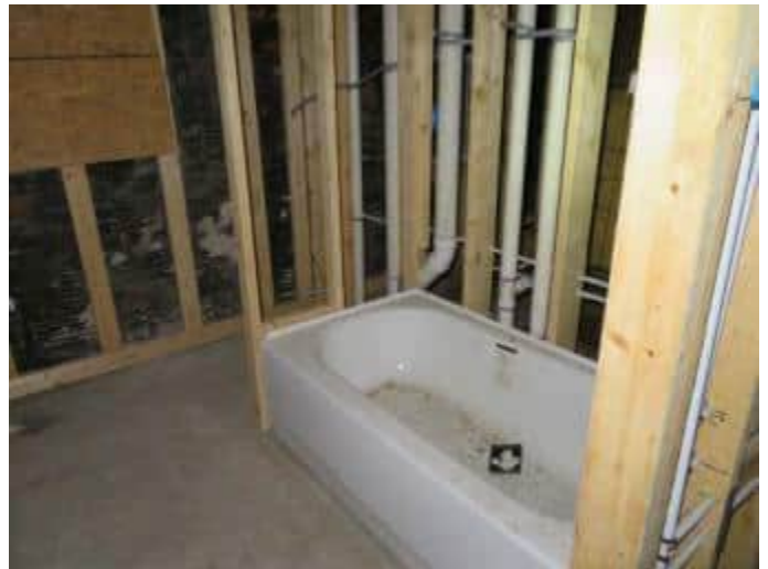
107. Repairs at fire damaged unit.
