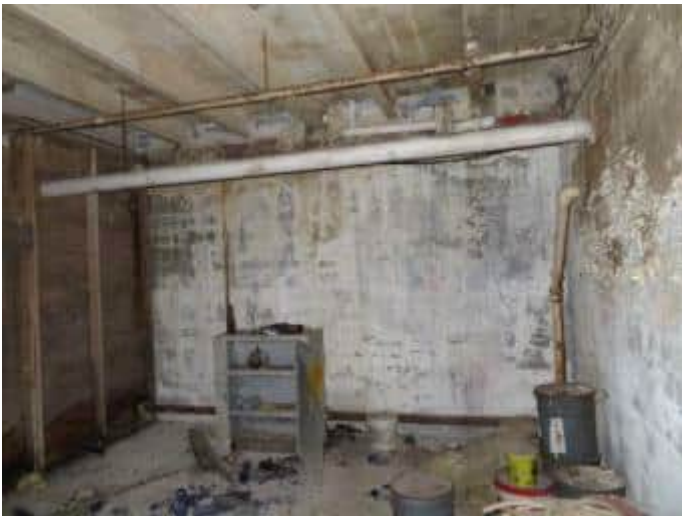
22. Interior view of basement area.
