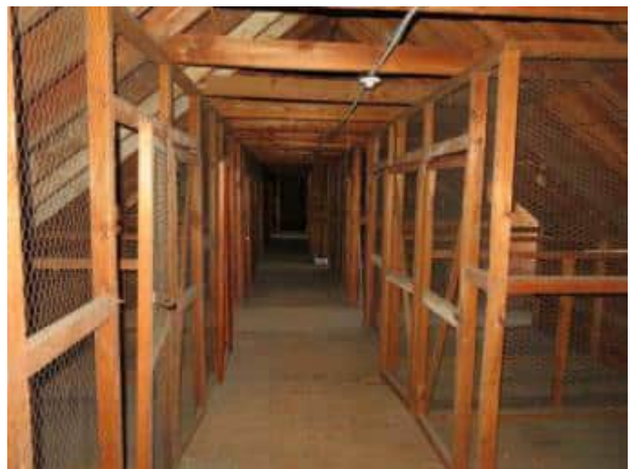
25. Wood framing at attic.
