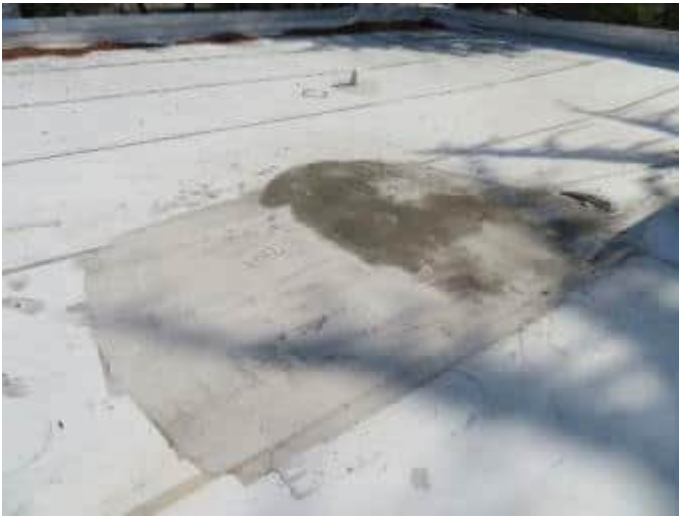
44. Area of prior repair at TPO membrane roofing.
