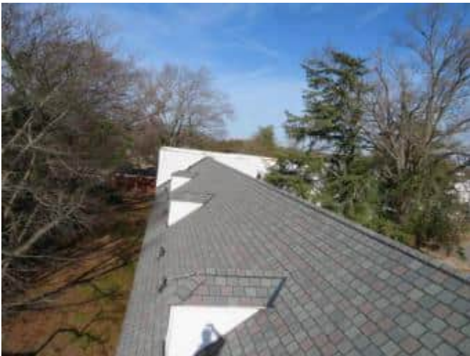
52. Pitched asphalt shingle roofing at center section.
