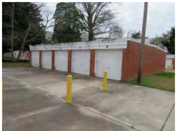
7. Typical parking garage building.
