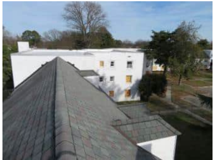
53. Typical condition of built-up roofing.
