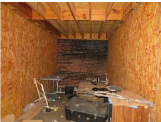
12. Interior of typical storage unit.
