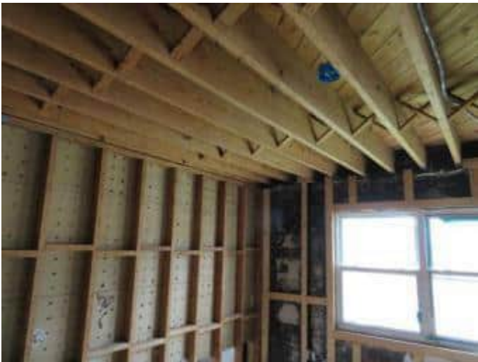
106. Repairs at fire-damaged unit.
