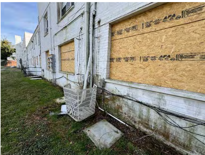
66. AC condenser unit removed from slab.
