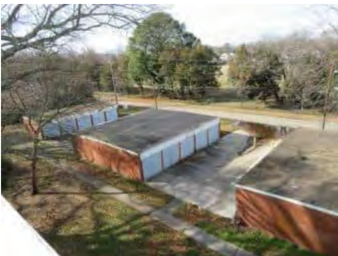
5. Parking garage buildings at the north side of the site (several have been converted to storage).
