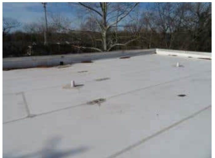
43. Low-sloped TPO membrane roof assembly at apartment building.
