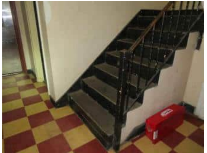
89. Common area stairwell finishes.
