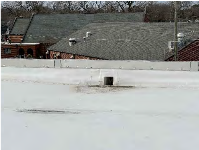
58. Roof scupper drain that discharges to downspout.
