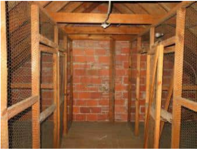
26. Wood and masonry framing at attic.
