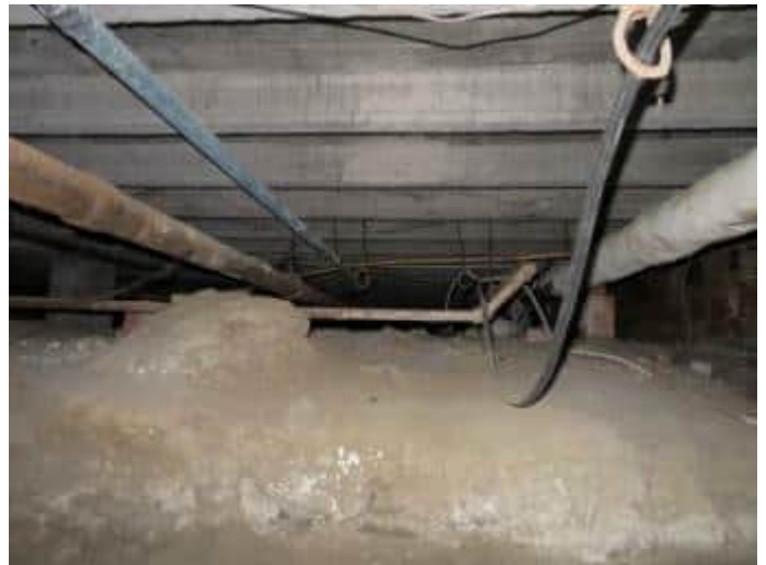
23. Crawlspace at apartment building.
