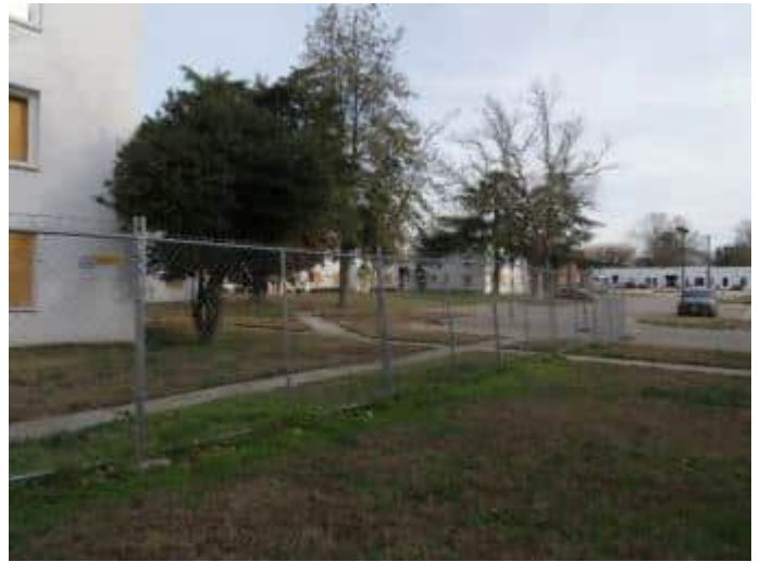
21. Temporary chain link fencing at perimeter of fire-damaged building section.
