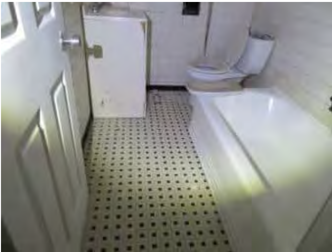
94. Dwelling unit bathroom finishes and fixtures.
