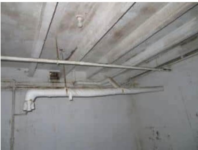
24. Concrete framing at first floor over basement area.
