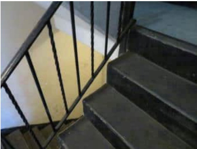
88. Interior common area stairwell.
