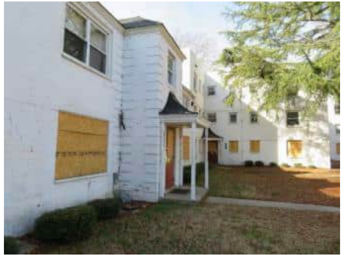
27. Exterior walls consist primarily of painted brick veneer with concrete elements.
