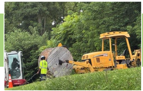
Wireline broadband infrastructure under construction in Bedford County.
